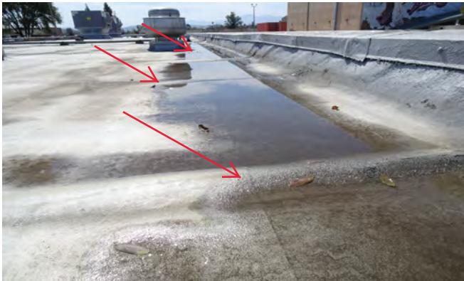
7.) View of ridging occurring at existing roof membrane.
