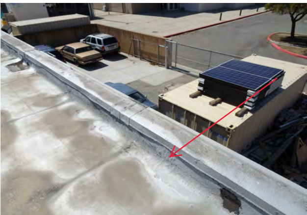
5.) Overall view of splits developing at parapet wall base flashing on the west section of building.
