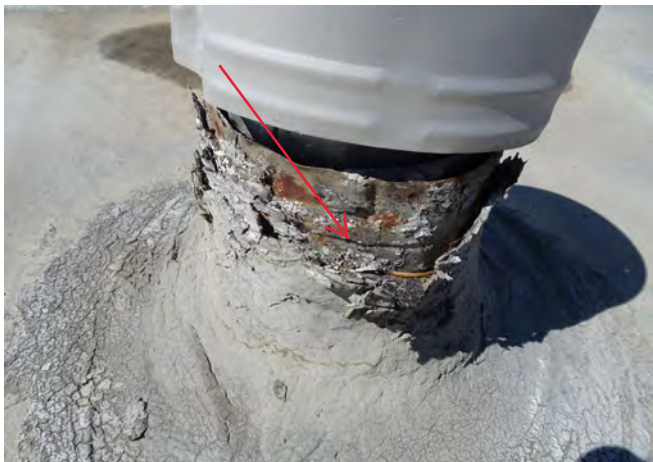
9.) Close up view of pipe flashing not sealed and exposed to the elements.
