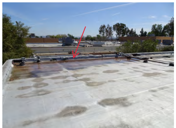
12.) Overall view of water ponding on the northeast corner of building.
