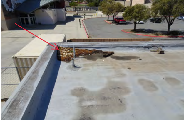
1.) Overall view of roof on the southwest corner of building. Debris accumulating along parapet wall base flashing.
