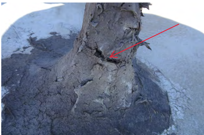
11.) Close up view of splits developing at mastic repairs.
