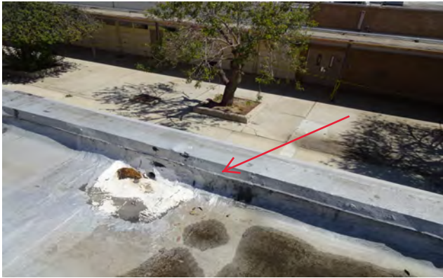
13.) Overall view of splits at roof scupper drain.
