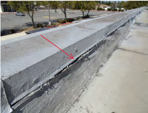
3.) Overall view of base flashing membrane not properly tucked under coping flashing. Base flashing exposed to the elements.
