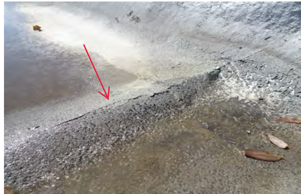
8.) Close up view of degrading roof membrane near wall base flashing.
