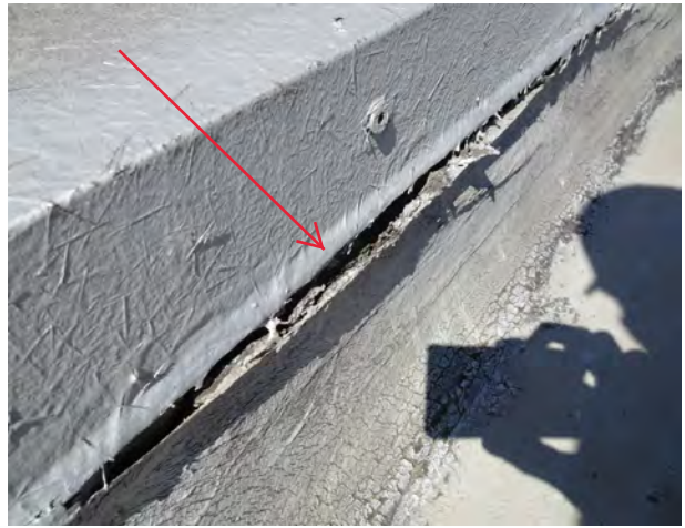
4.) Close up view of exposed base flashing on the west section of building.
