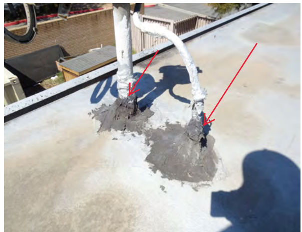
10.) Overall view of splits developing at mastic repairs.
