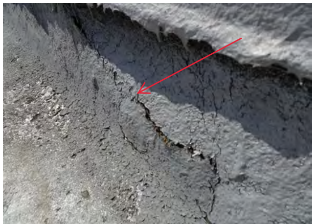
6.) Close up view of split occurring at base flashing membrane on the west section of building.
