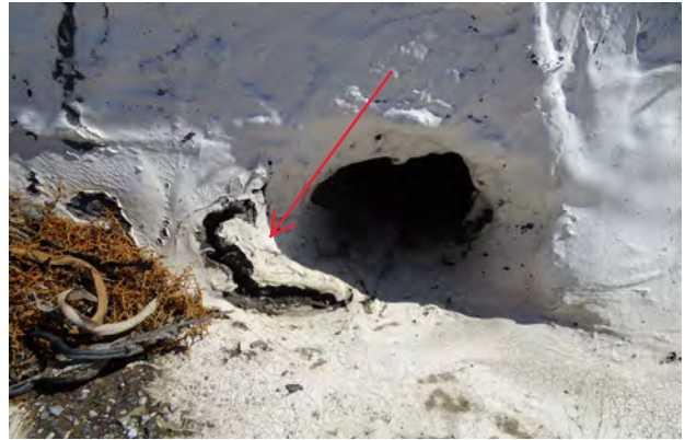
14.) Close up view of split occurring at roof scupper drain.
