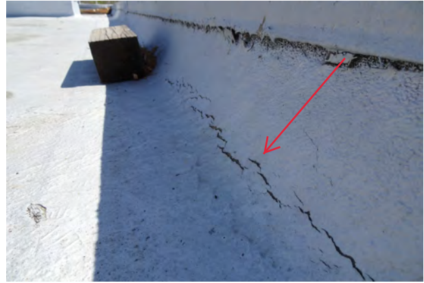
2.) Close up view of splits developing along parapet wall base flashing membrane.
